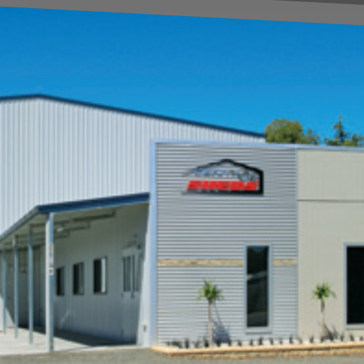
Central Vic Sheds is built on a solid foundation of quality and service
